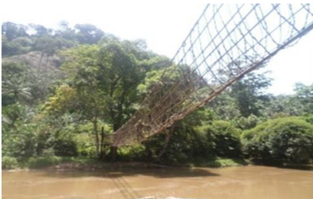
a) Existing rope bridge at Ollorunti river
