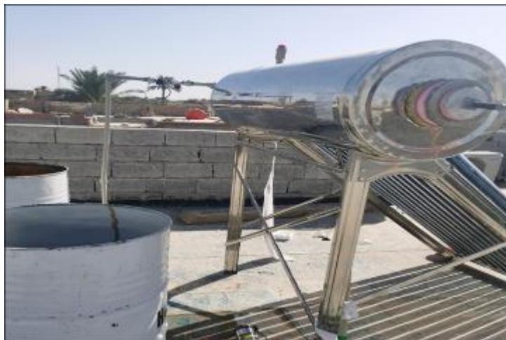
Figure 1 Evacuated tube solar collector system
