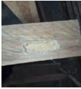
Plate 5: drilling the mortise and tenon joint
