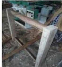
Plate 6: coupling the frame
