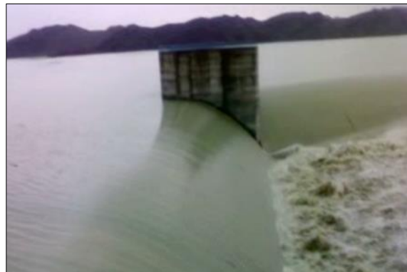
Figure 2 Spillway of the Pishin Dam with bankfull flow during flash flood in the stem of Sarbaz River 2020
