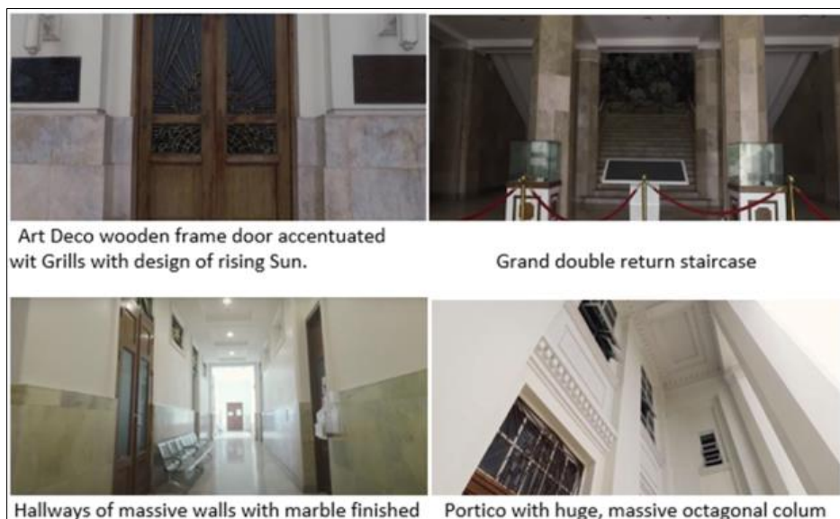
Figure 7 Bulacan Provincial Capitol Architectural Art Deco Features source: "Ako Ang Kapitolyo" - SINEliksik Bulacan Documentary Special (Proyekto ng: United Architects of the Philippines Barasoain Chapter)
