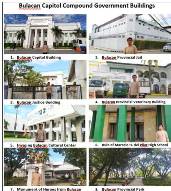
Figure 22 Other Heritage Structures at the Bulacan Capitol Compound
