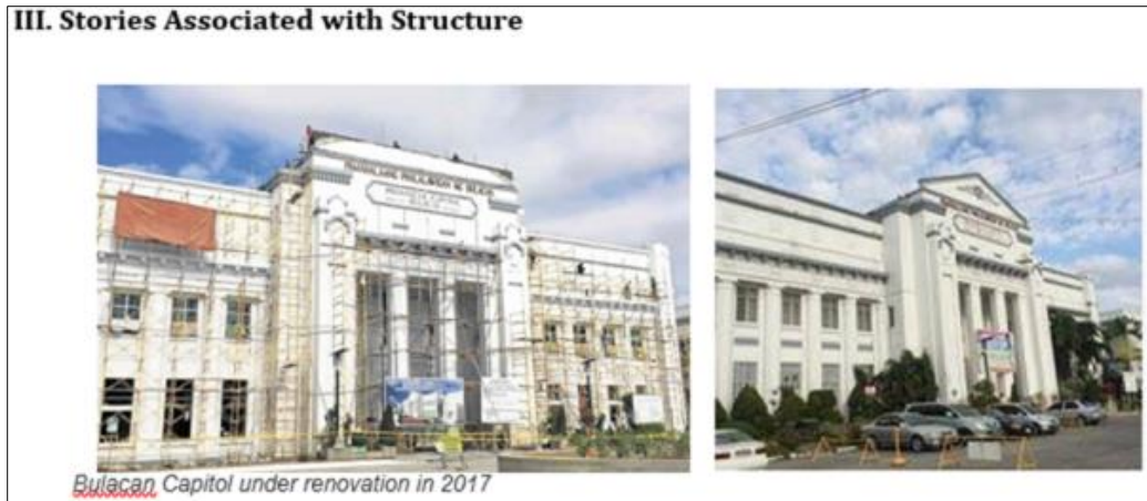
Figure 17 Bulacan Capitol under renovation in 2017 (Photo credit: Melanio Martinez Jr.)
