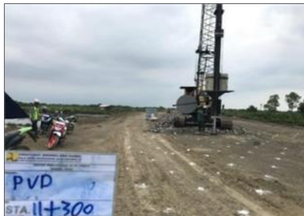
Figure 10 PVD installation process
