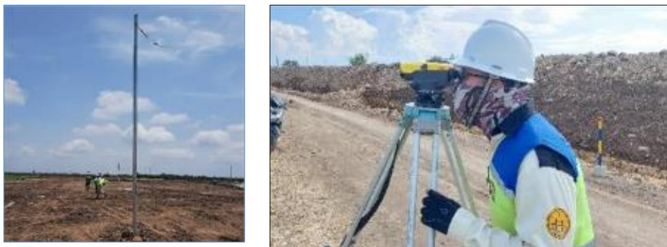
Figure 6 Monitoring of Land Subsidence with Settlement Plates
