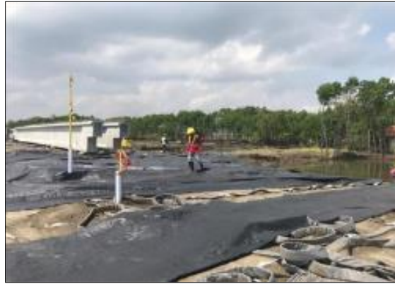
Figure 11 Process of installing PHD, sand and non-woven geotextiles
