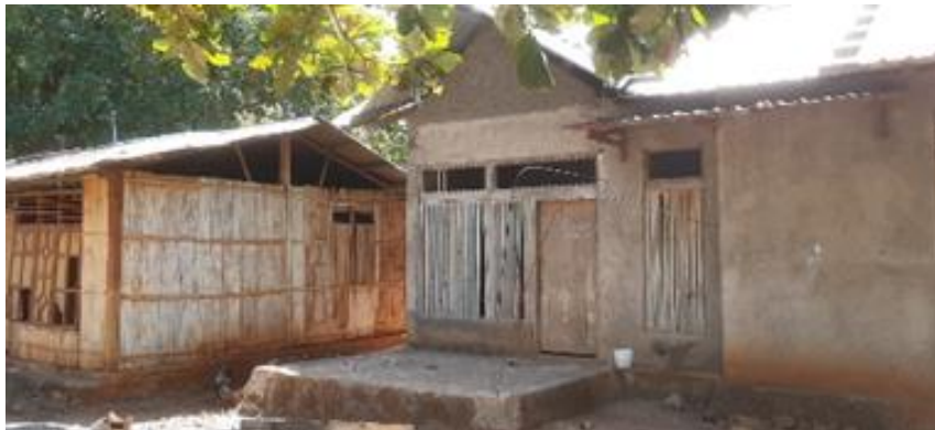
Figure 1 One of the residences with loose walls in Sikka Regency (source: Personal Documentation, 2023)
