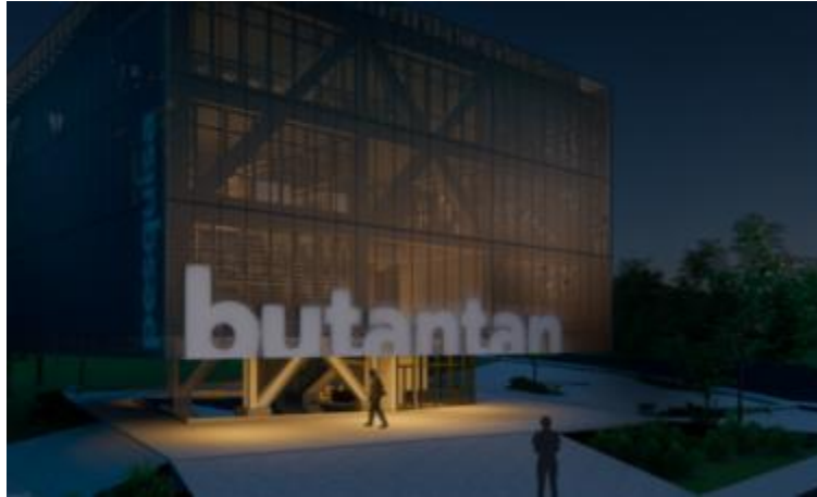
Figure 5 Night image of the technical block.
