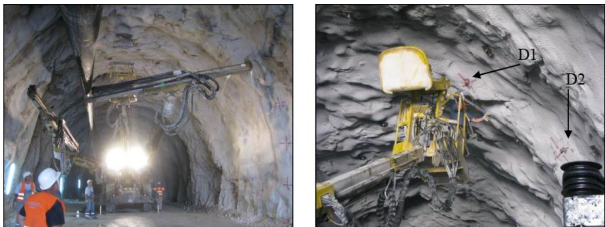
Figure 11 Drilling boreholes for installing anchors and initiating signals on the anchor [9]
