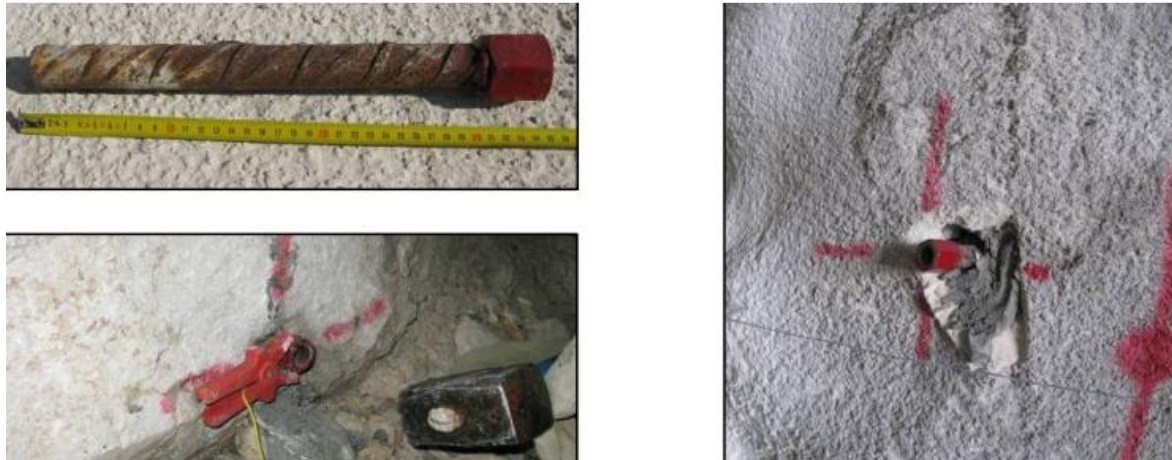
Figure 12 Anchor before installation, after installation and during measurement [9]
