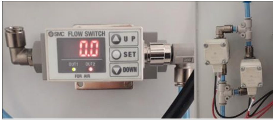
Figure 6 Flow controller. PF2A series flow switch - PF2A710-01-67 supplied by SMC company, with high precision adjustments in the range of 0.1 l/min. ON/OFF electric valves. Process Directional Valves VX2 - VX210BA manufactured by SMC supplier, with ON/OFF type relay contact activation. This type of control valve was chosen so that the system could operate automatically and autonomously. Source: From the author (2021)
