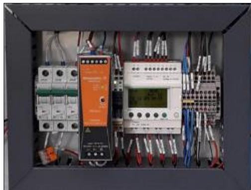
Figure 2 PLC – programmable logic controller. It is digital electronic equipment with hardware and software compatible with industrial applications. Source: From the author (2021)
