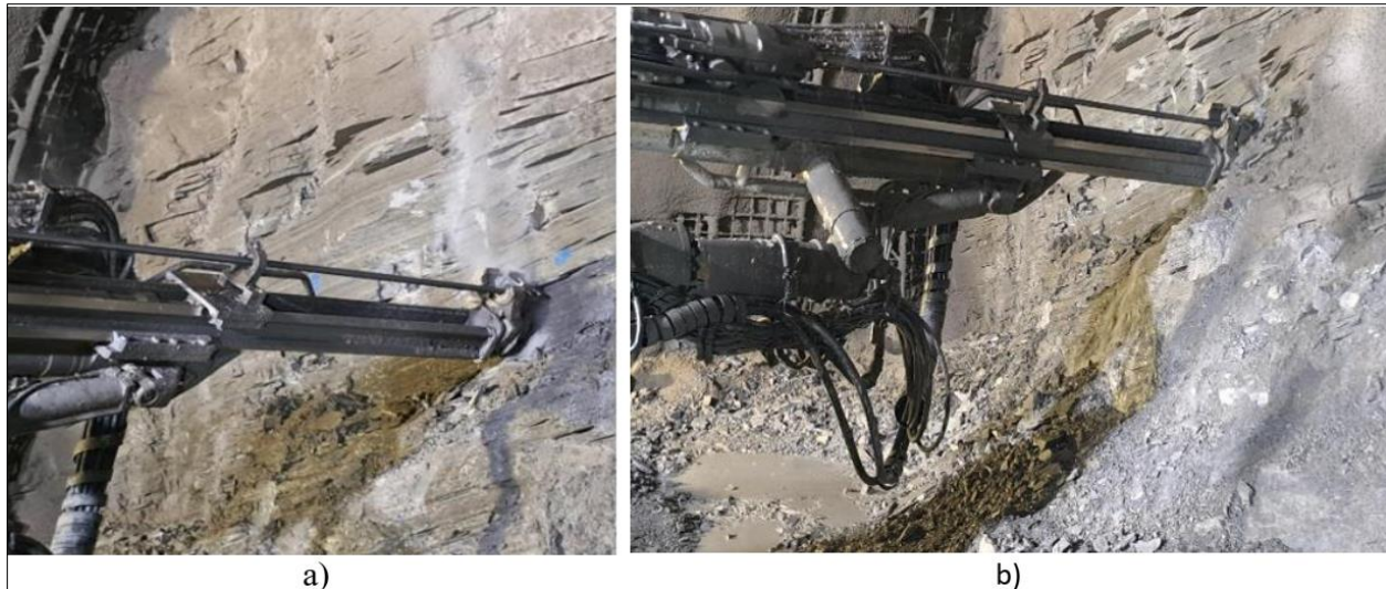
Figure 8 Presentation of drillholes drilling: a) dry process and b) wet process
