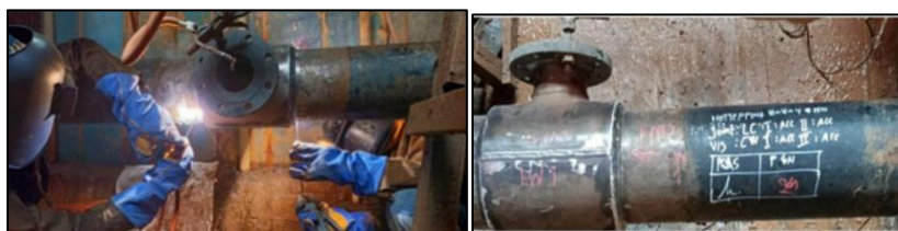
Figure 2 Split Tee Welding Process and Post-Weld Visual Inspection
