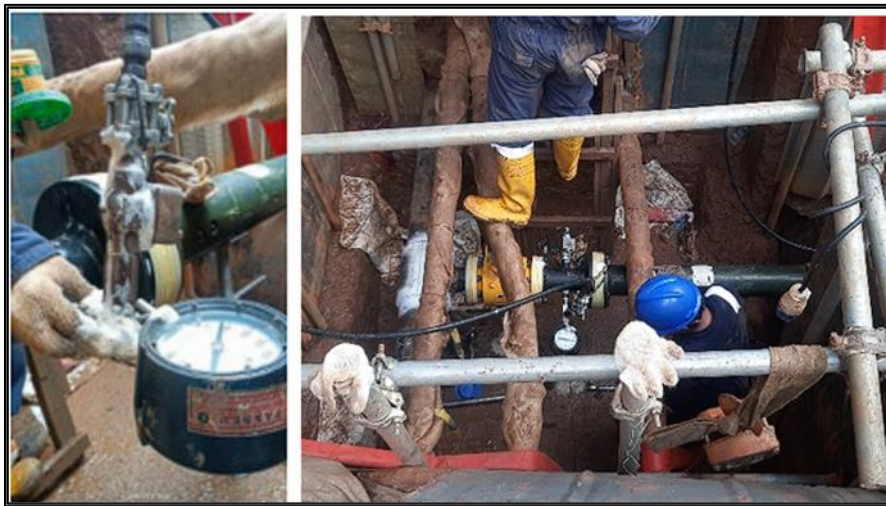
Figure 3 Leakage test
