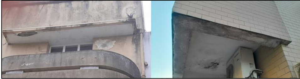
Figure 1 Examples of buildings with damage caused by hygrothermal stresses
