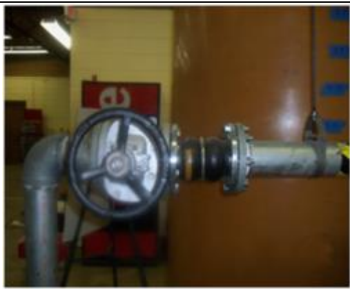
Figure 5 Outlet Valve
